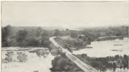
3RD STREET BRIDGE OVER DEEP RIVER
